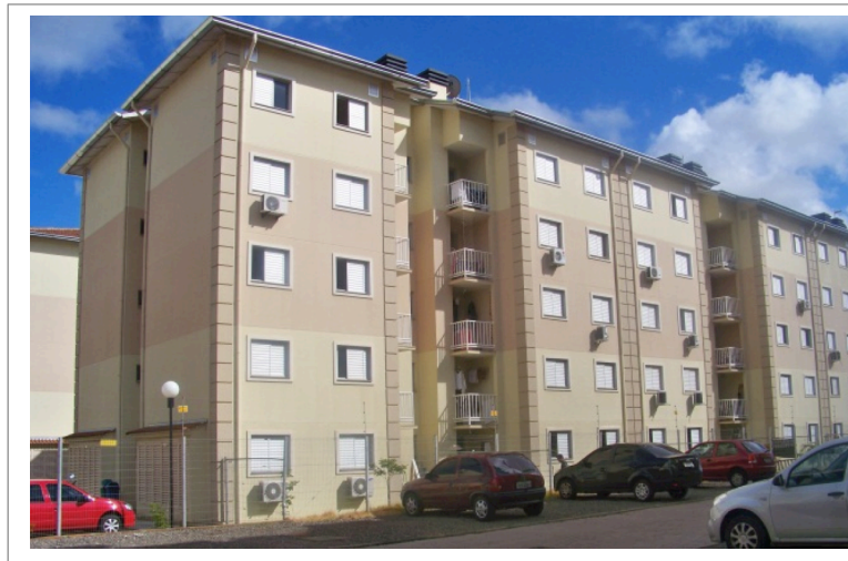
Figure 2. View of a finished block of flats. Source: authors
