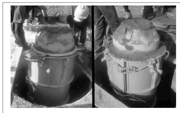
Figure 2. Densification of concrete by the vibration production system
