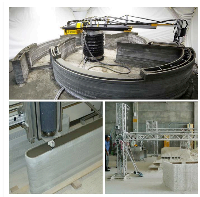
Figure 1. 3D printed construction technologies (above: concrete printing; below left: contour crafting; below right: D-Shape printing. Source: (Ghaffar et al., 2018) and (Ma et al., 2018)
